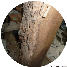
柱の腐朽
